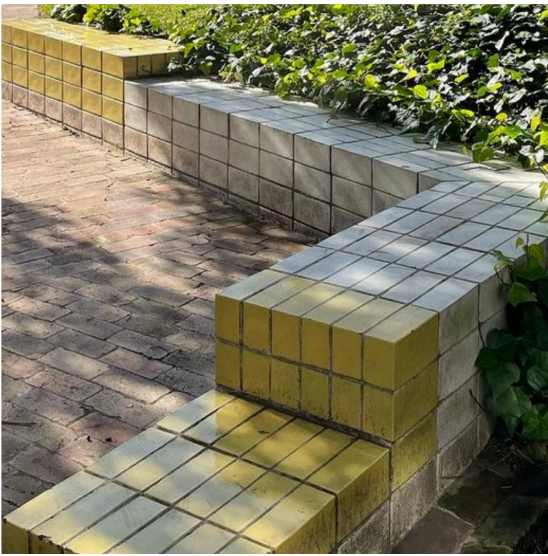
Low brick retaining & seating walls <500mm height
