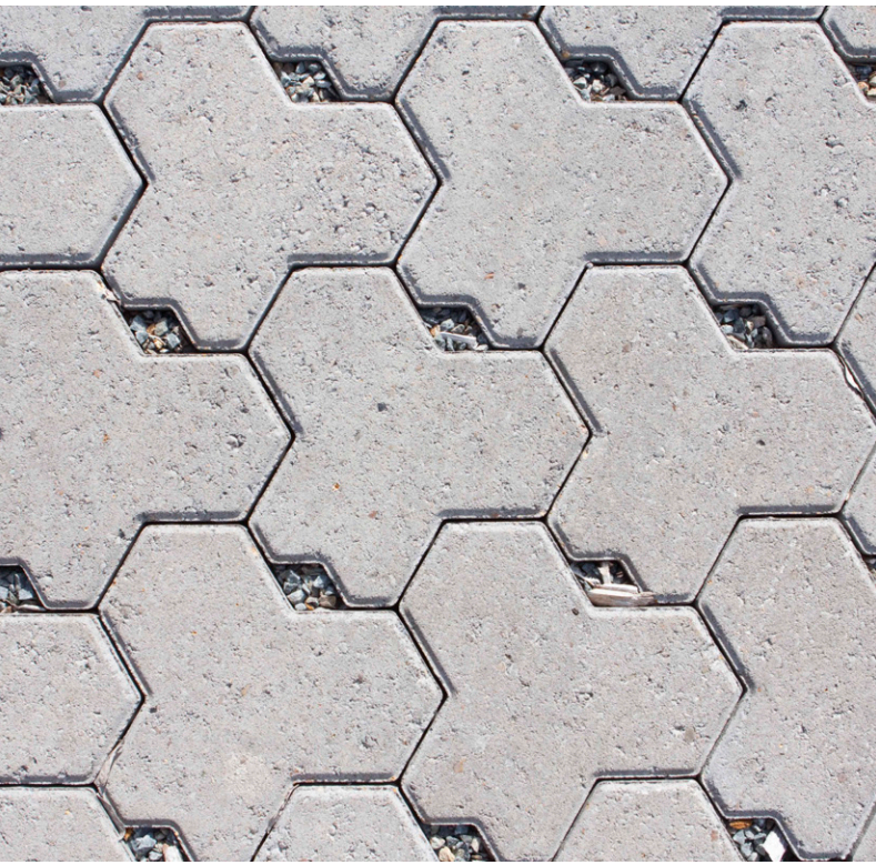
Permeable unit paving (shot blast finish)
